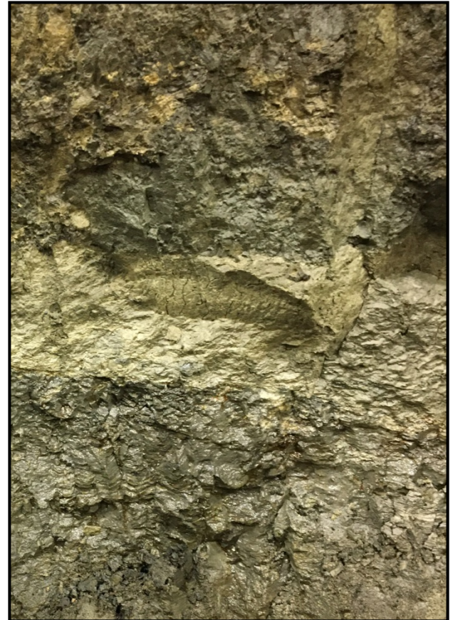
PHOTOGRAPH #2: Oily surface on the soil at S27 at approximately 2.0 metres below grade.
